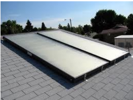
Figure 1. Solar Water Heater Panels (NREL)
